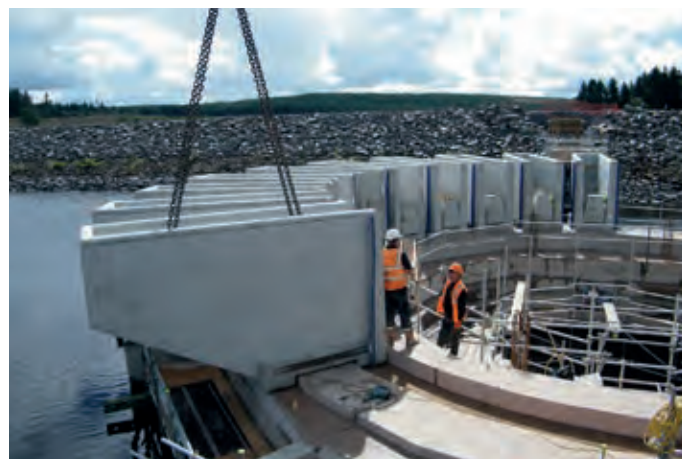
Construction of the new weir at Black Esk Reservoir
