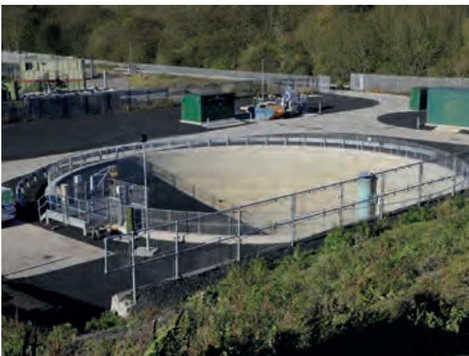
The storage tank at the Cowdenbeath Wetlands scheme
