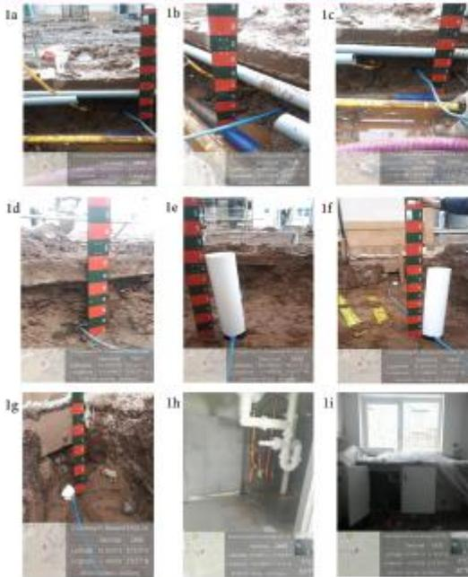
**1st Photograph Far-side 1a** A photograph showing the line of the communication pipe from the far-side excavation to the near side, excavation. The communication pipe must be at 90° degrees from the main to the Boundary stop valve.
