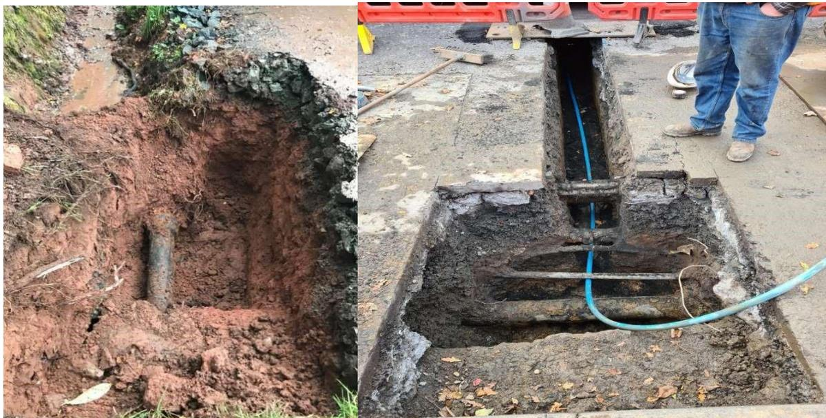
Exposed water main for connection – excavation should be approx. 1m x 1m and 150mm clearance below the main to allow for the connection. A measuring stick /tape should be used to show the depth of the main to the finished ground level to allow for safe access/egress from the excavation.
