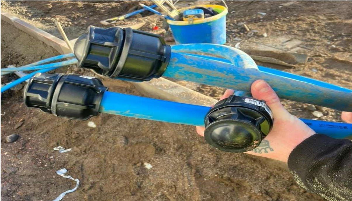
The supply must be capped off with either a plastic cap or a Philmac fitting and must be shown in the photo above.
