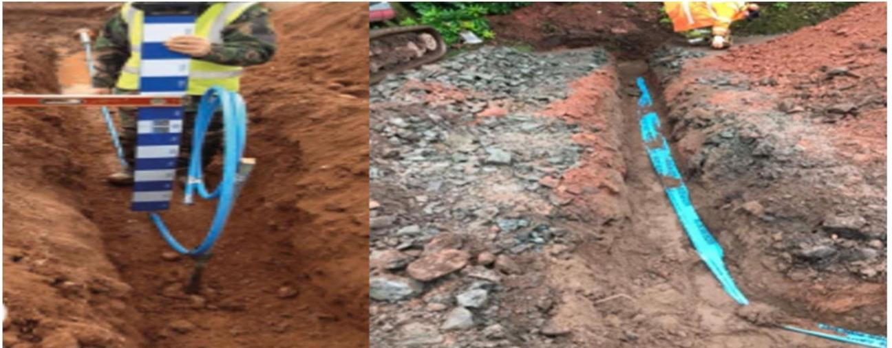
Track with sand, pipe and marking tape laid above. This should be a minimum depth of 750mm, and Marker tape should be laid at a 100mm-300mm above the supply pipe for the whole length of the track.
