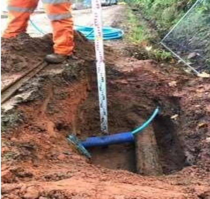
Example of a far side connection (Road Crossing) showing the supply going through a 100mm BLUE Duct at a minimum depth of 750mm.
