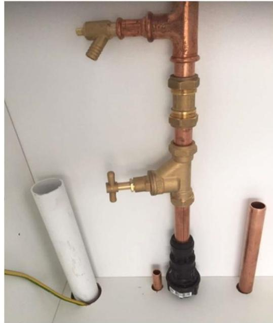
Internal fittings installed – hand control, double check valve and drain off.
