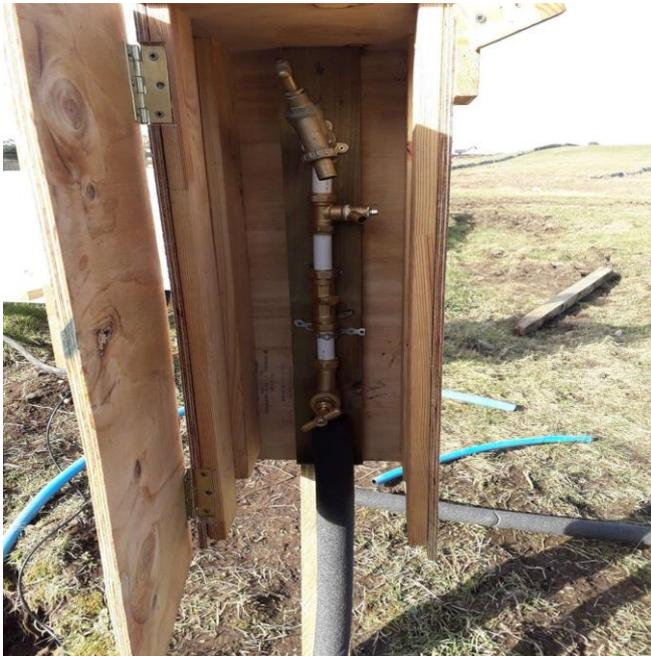
If setting up a standpipe for building water – the supply should be insulated above ground and have a hand control, double check valve, drain off, bib tap and should be in a secure box.
