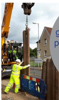
The sheets are driven into the ground to secure the pit for excavation and prevent ground movement. **Very Noisy.**
