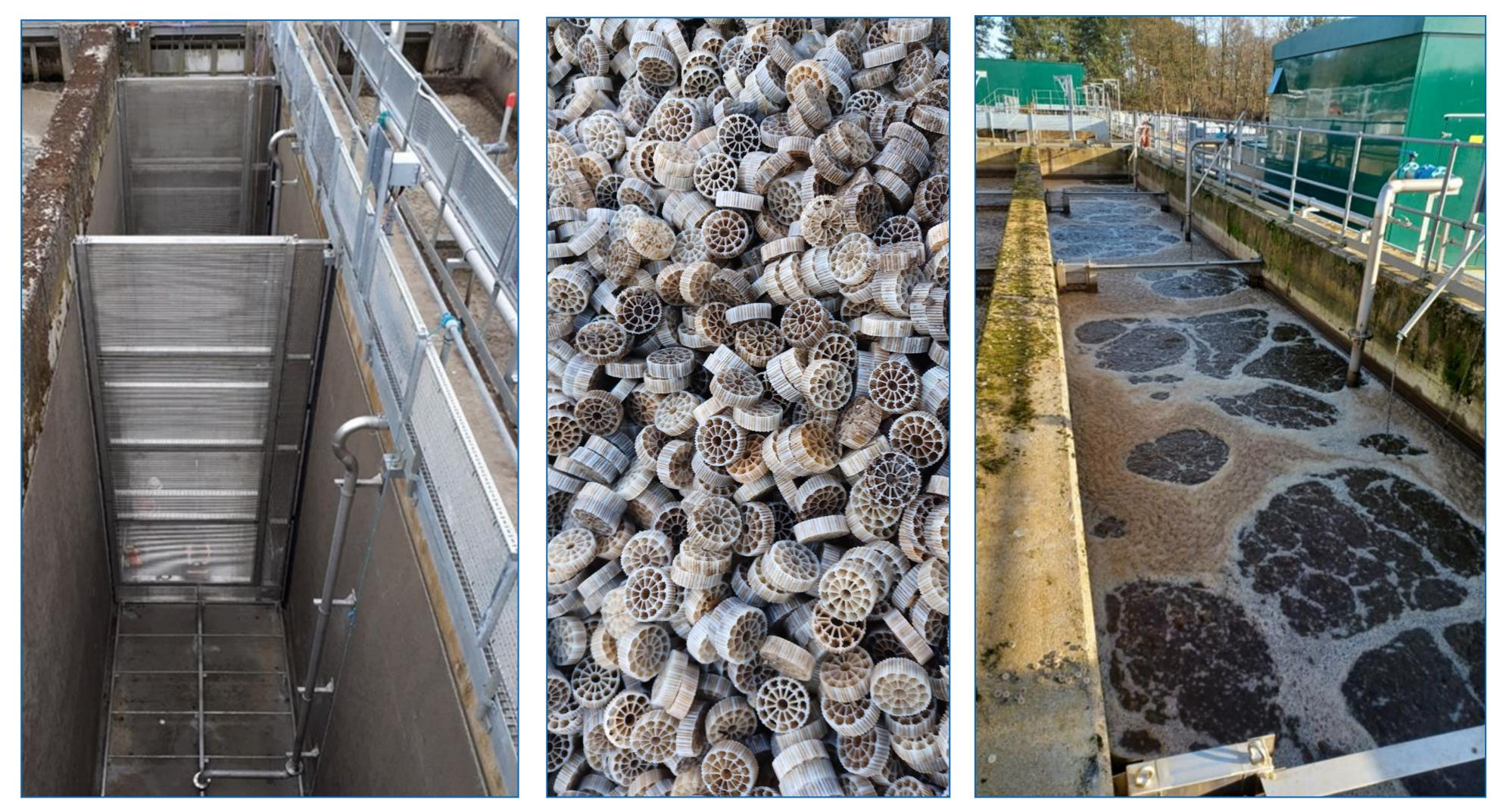
• Left: the deep aeration lanes and the screens which divide them into cells before entering operation. Middle: the plastic biofilters which are associated with the IFAS technology and host communities of bacteria to rapidly break down nutrients in the waste water. Right: the IFAS aeration lanes in operation.
