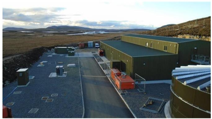
An example of a transportable water treatment unit which has been installed by Ross-shire Engineering in Lochmaddy, Western Isles. The proposed Water Treatment Works for Peebles will include buildings which will \_be pre-fabricated and delivered to the site from Ross-shire Engineering's factory in Muir of Ord.
