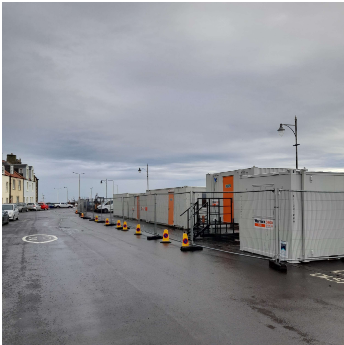
Image: Current Site Compound on Mid Shore
