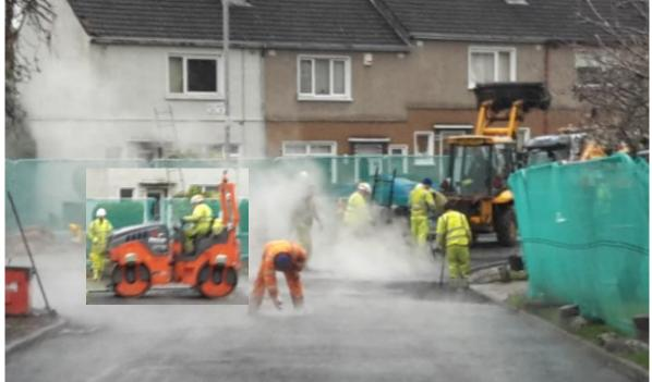
8) The excavated area is backfilled and reinstated. The grassed area (in the red box to the left) will landscaped then seeded.
