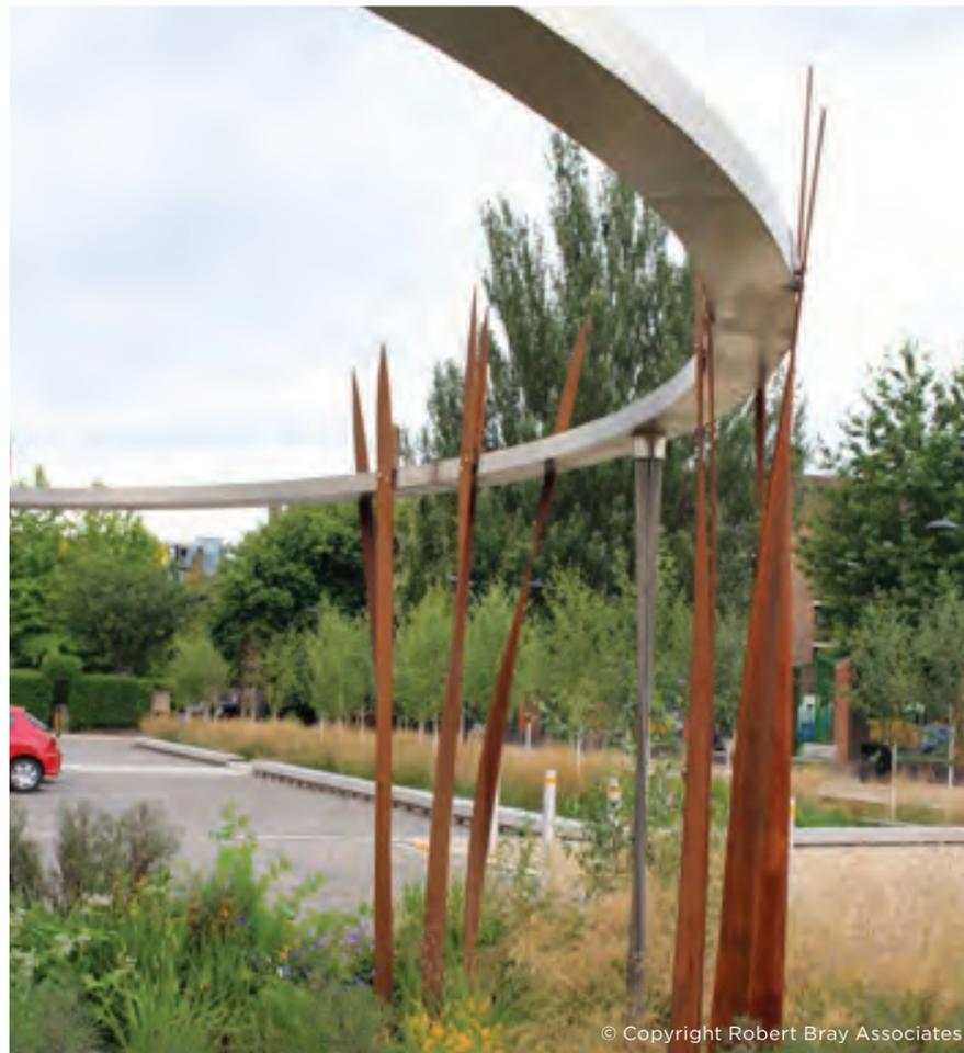
fig. 47: Surface drainage from the roof incorporates sculpture
