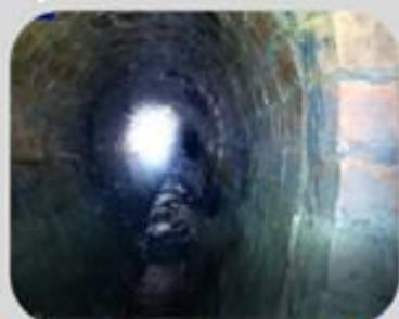
The sewer is accessed from a manhole and a camera survey is undertaken
