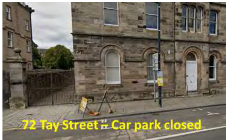
Image: Private car park at 72 Tay Street closed.
