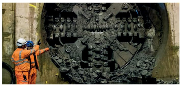
Daisy the Driller is pictured after its cutting head 'broke through' at the end of the tunnel in Queen's Park, Glasgow
