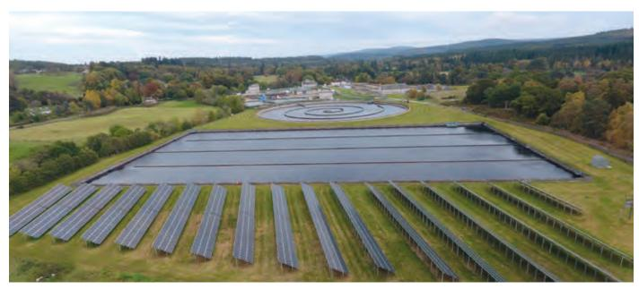
Photovoltaic solar panels at Invercannie Water Treatment Works
