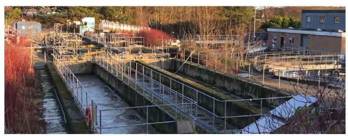
Ellon Waste Water Treatment Works showing the aeration lanes where IFAS will be deployed
