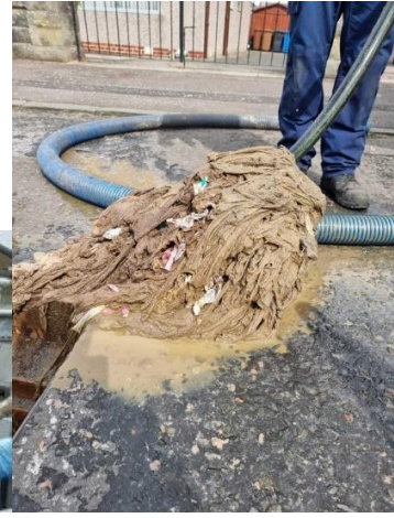
One of our 36,000 sewer blockages per year being cleared
