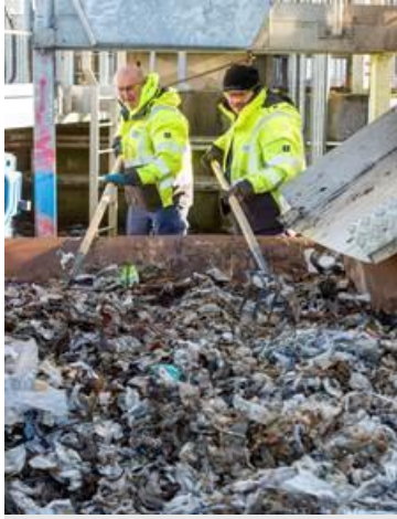
Inappropriately flushed items screened out at the wastewater treatment works
