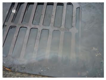
Oil sheen visible on the water surface at this blocked drain
