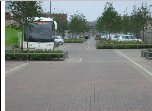
Photo 2. Permeable block paving on the site
