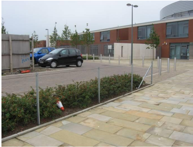
Photo 6. . Different Types of Paving Used on Site.
