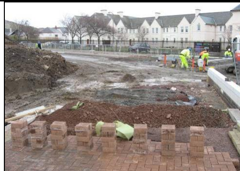
Photo 4. Road Construction Type M1 in Progress
