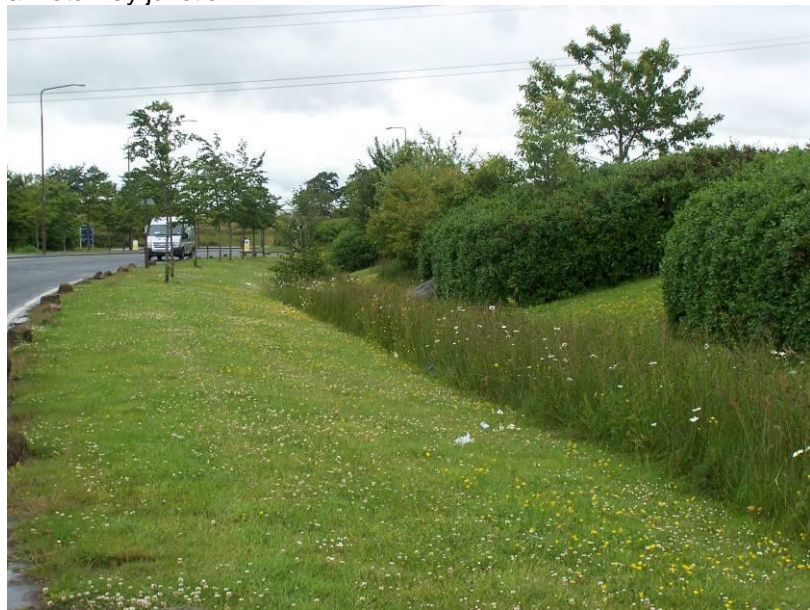
Photo 9. Filter Strip and Swale
