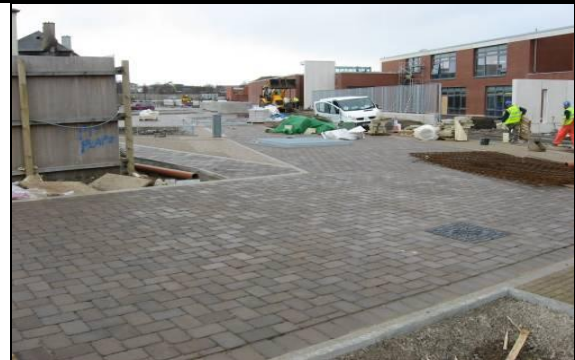
Photo 5. Road Construction Type M2 Completed
