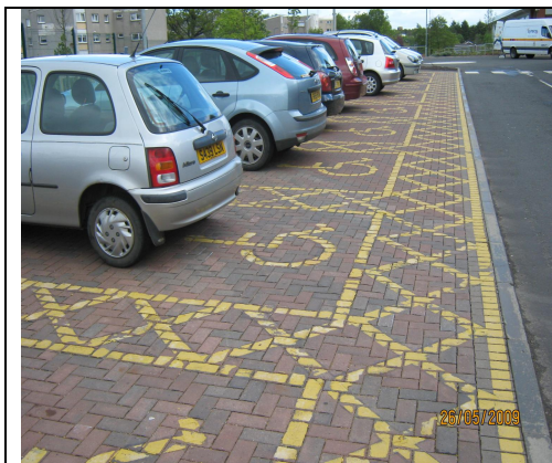
Photo 7. Permeable paving at disabled parking spaces
