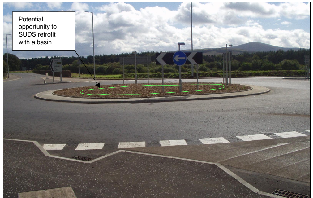
Figure 5.4 SUDS Retrofit in Roundabout Island, Lanark
