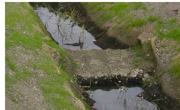
Check Dam to control flow velocity
