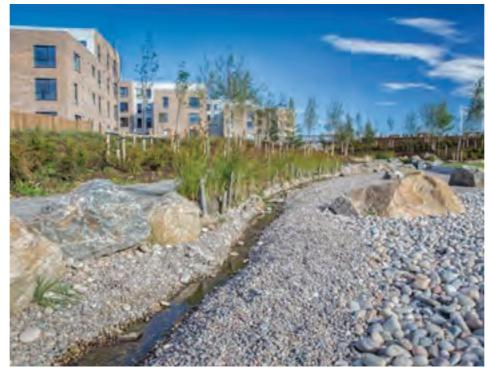
fig. 51: The Cults Burn: designed to accommodate fluctuating water levels
